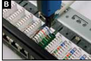
Terminate wires using Linkbasic tool (P/N: TLA01) or equivalent.
