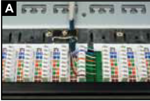
Insert each wire into the appropriate channel.
