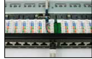
Insert the jack into the correct mounting location properly.
